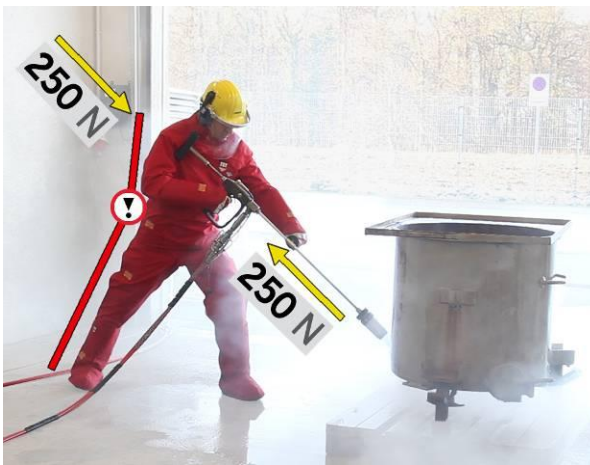
Manual blasting gun work
