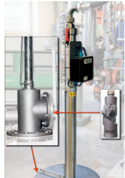
Gastight cleaning system with water/air driven lance
